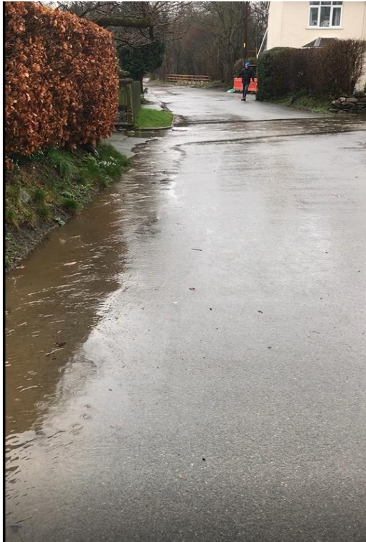
Figure 6: Initial floodwater overtopping from Afon Ceidiog near Plas Estyn. Source: Resident
